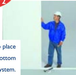
The first element is lifted into place and fastened to the profiled bottom rail using a special locking system.
