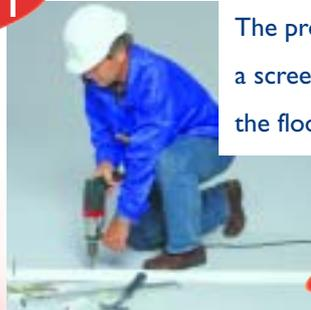
The profiled bottom rail is fixed onto a screeded floor base. It is fastened to the floor base using special bolts.
