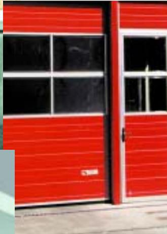
There are special rails in GRP for adding entrances and doors. Windows with GRP frames compatible with Beet walls can be supplied.
