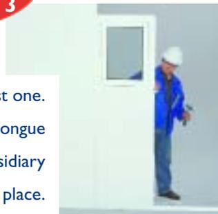
The next element is positioned beside the first one. The elements fit into each other on a tongue and groove basis. Pre-assembled subsidiary elements for windows, etc are fitted into place.
